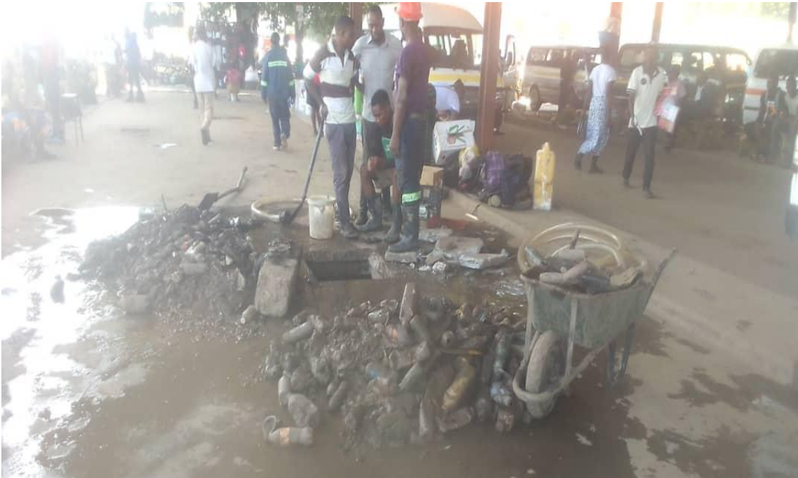
Figure 4: Shows the blocked drainage in intra bus station – Kabwe (Source: engineering Department - Kabwe Municipal Council)
