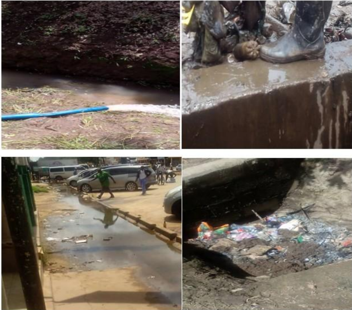
Appendix 2: Shows unblocking drainage system in different parts of Kabwe District
