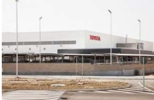
Toyota plant at Illescas (Toledo) - Spain
