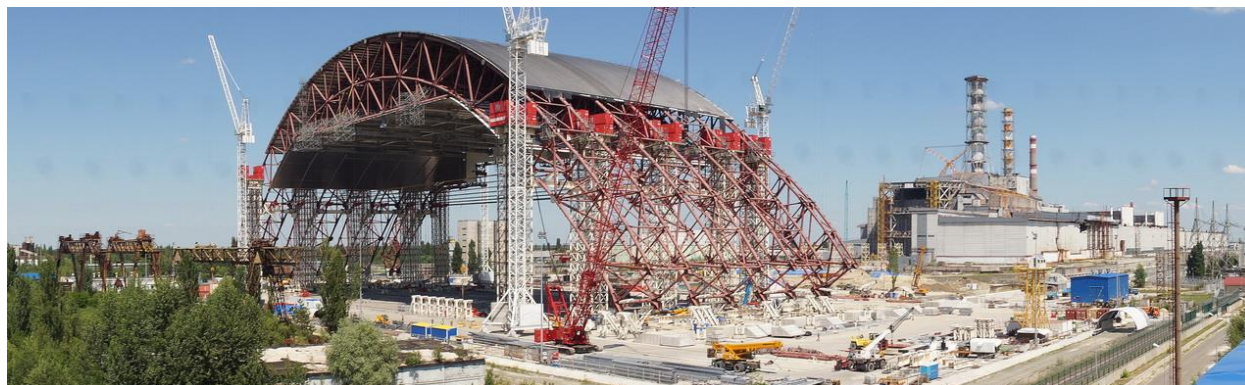
After 2-nd lift of eastern section on NSC Arch
