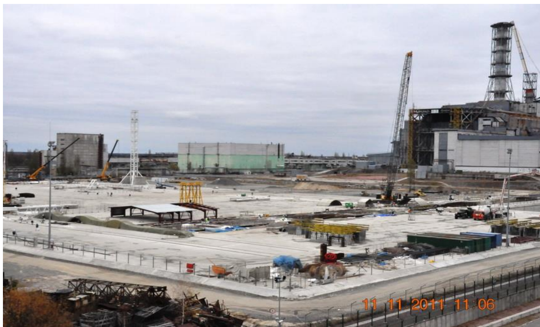
Platform for Arch assembly, November 2011
