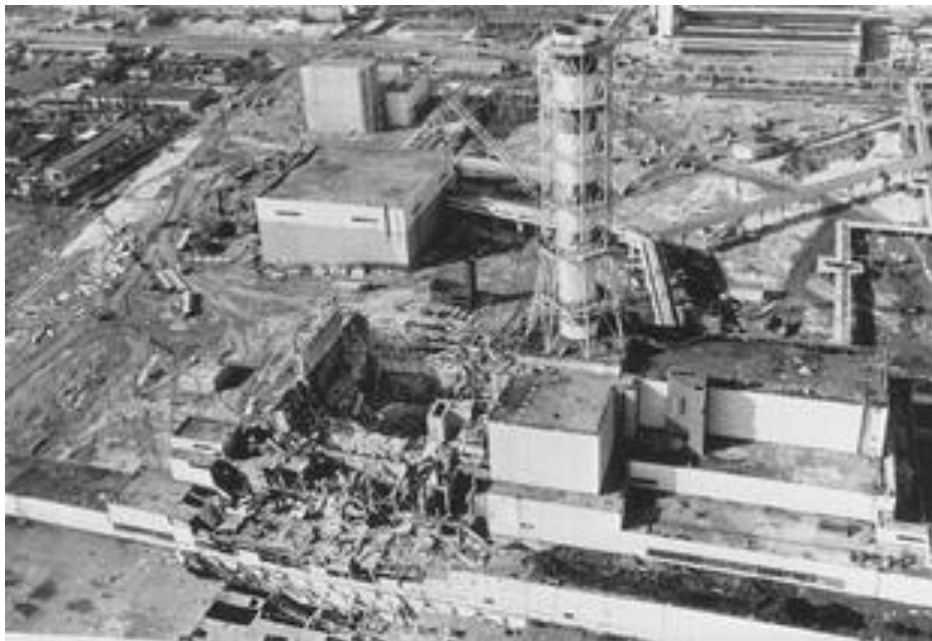
The destroyed 4th power unit of the ChNPP, April 1986.
