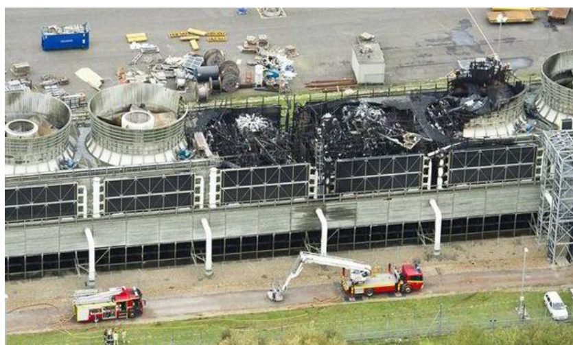
Aerial view of the damaged Didcot Power Station
