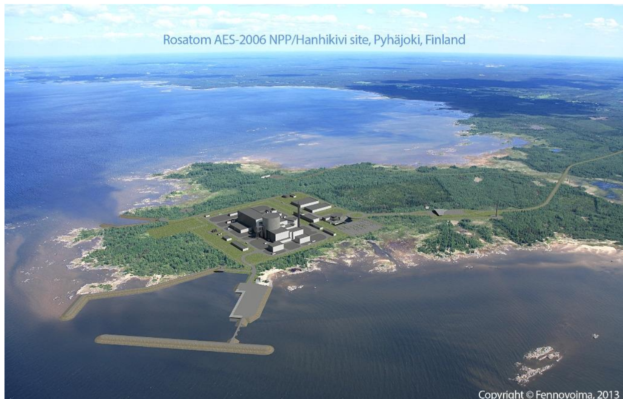
An illustration of completed Hanhikivi 1 site (photo courtesy Fennovoima)
