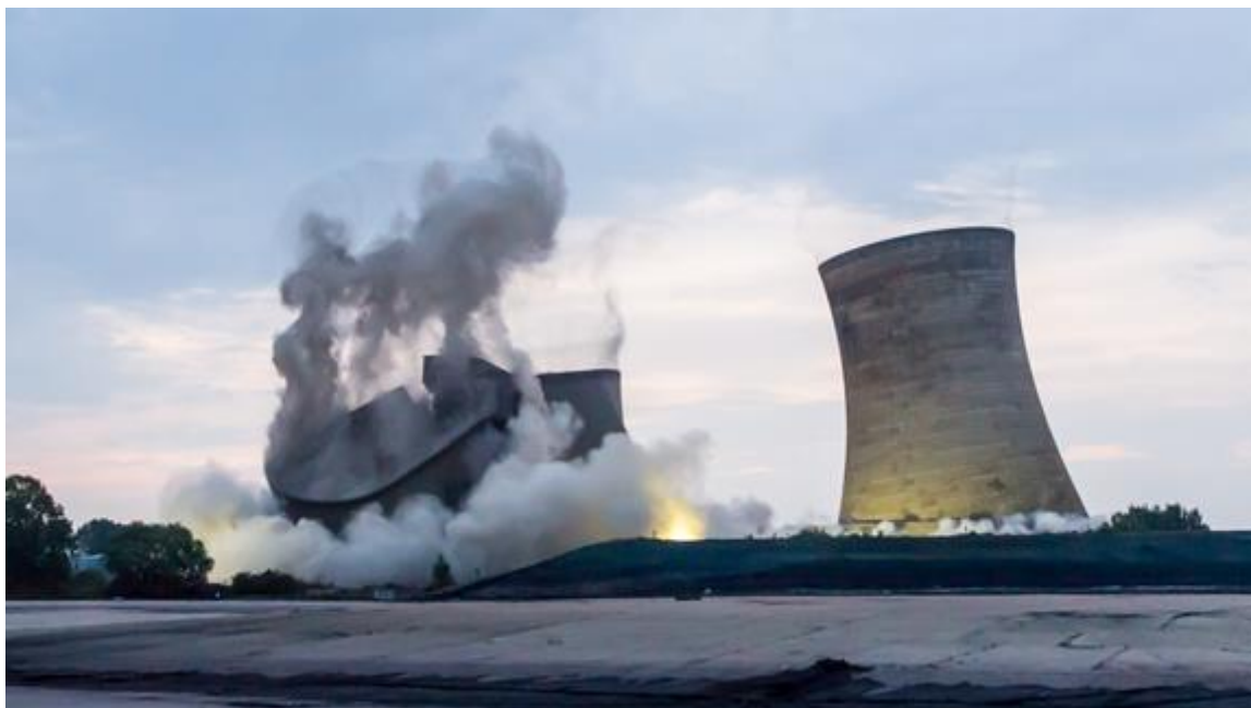
Cooling towers demolished July 2014 Photo courtesy npower
