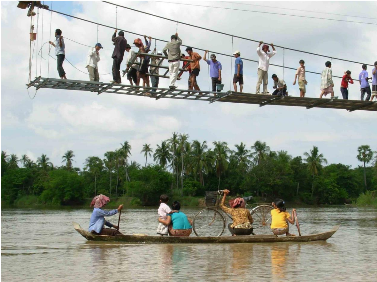
Bridge building at Koh Krosang, Pursat, Cambodia
