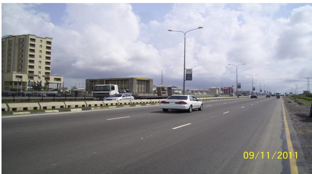
Fig 2: Rehabilitated & Upgraded Section of the Lekki-Epe Toll Road. Source: Author (2011)
