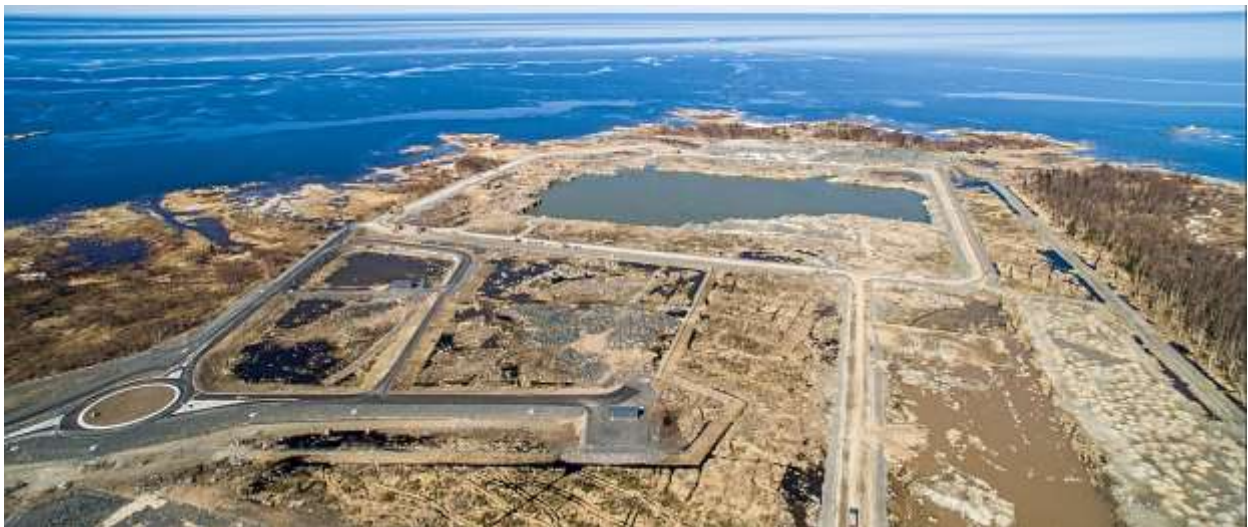
In the photograph: Aerial view of Hanhikivi 1 site (photo courtesy Fennovoima)
