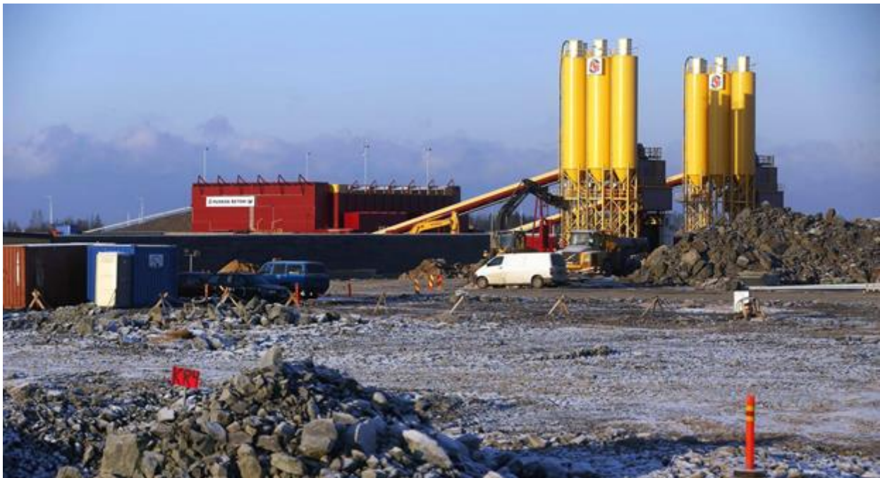
In the photograph: The Hanhikivi construction site (photo courtesy Pekka Fali)
