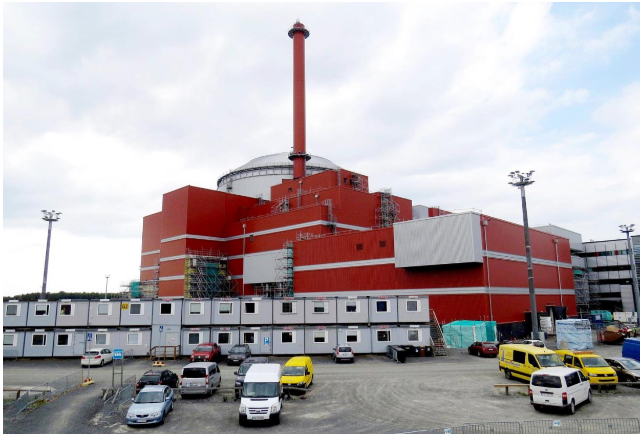
In the photograph: Olkiluoto 3 construction site (photo courtesy Lefteris Karagiannopoulos)
