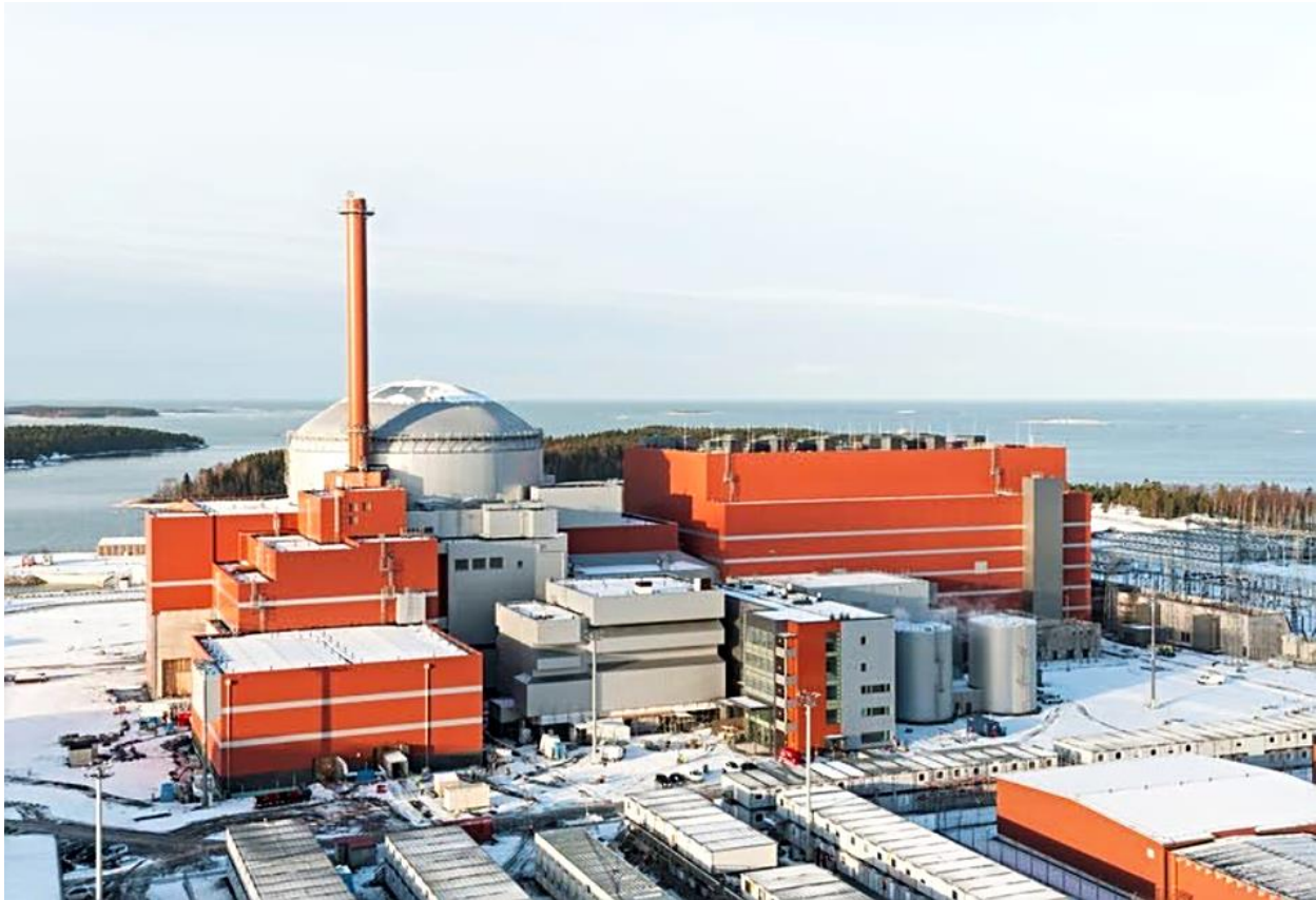
In the photograph: Olkiluoto 3 construction site (photo courtesy TVO)
