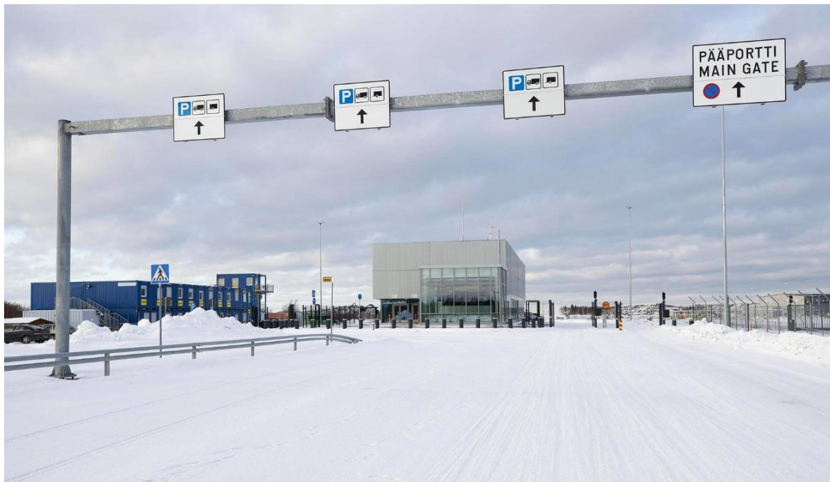
In the photograph: The Hanhikivi construction site main gate (photo courtesy Pekka Fali)
