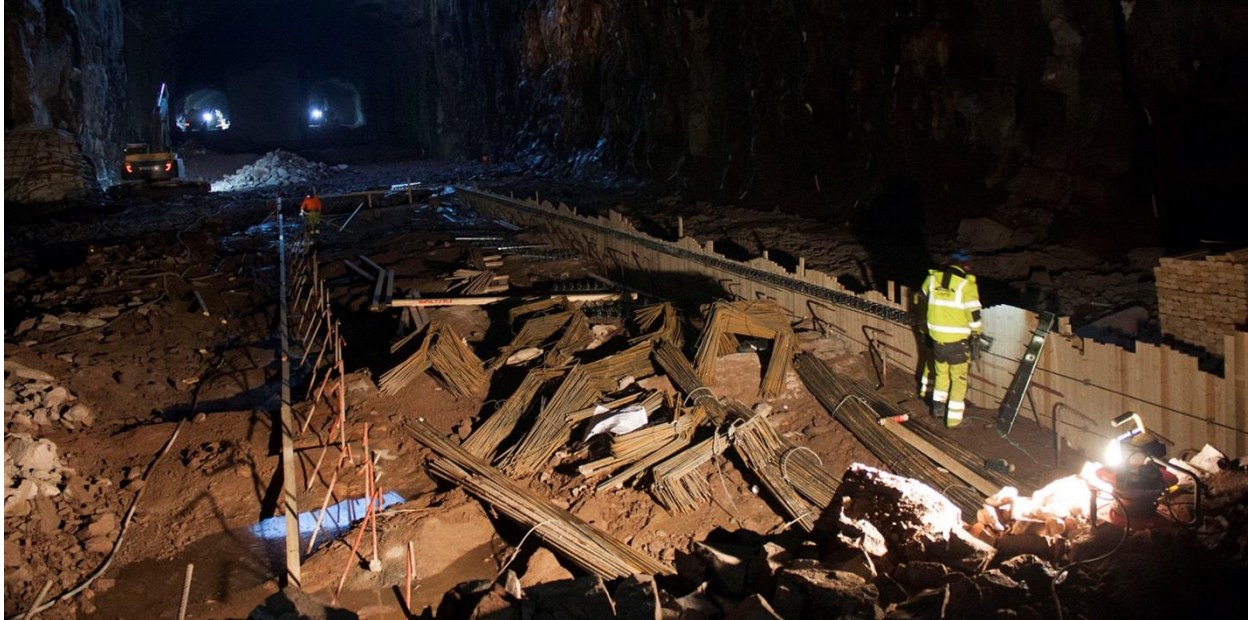
Kivenlahti station construction under way (photo courtesy Länsimetro)
