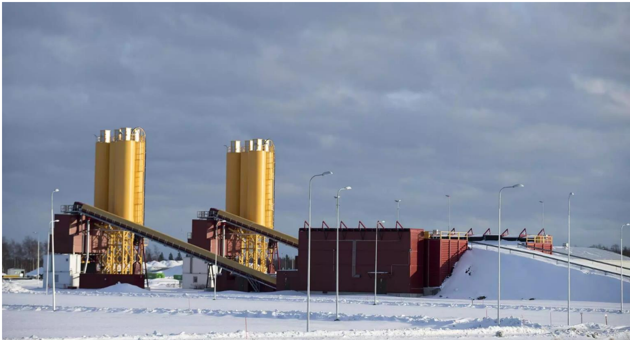
The Fennovoima construction site at Hanhikivi (photo courtesy HS / Pekka Fali)
