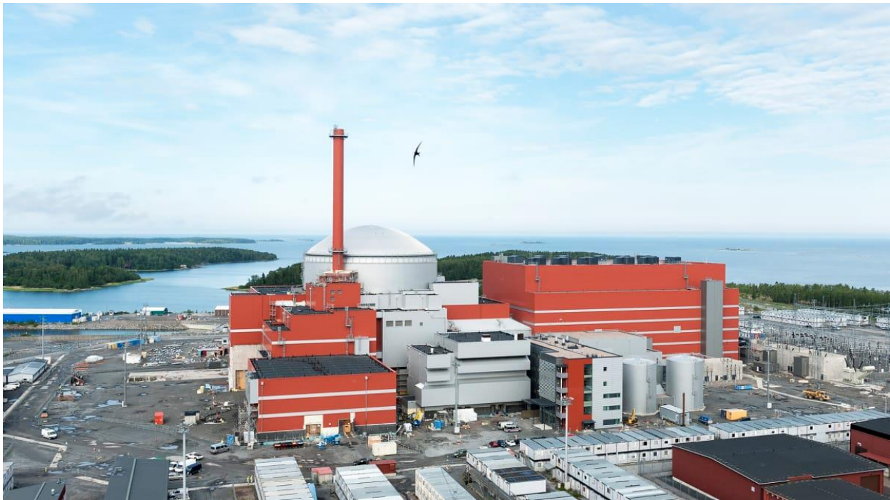
Olkiluoto 3 almost complete (photo courtesy TVO)
