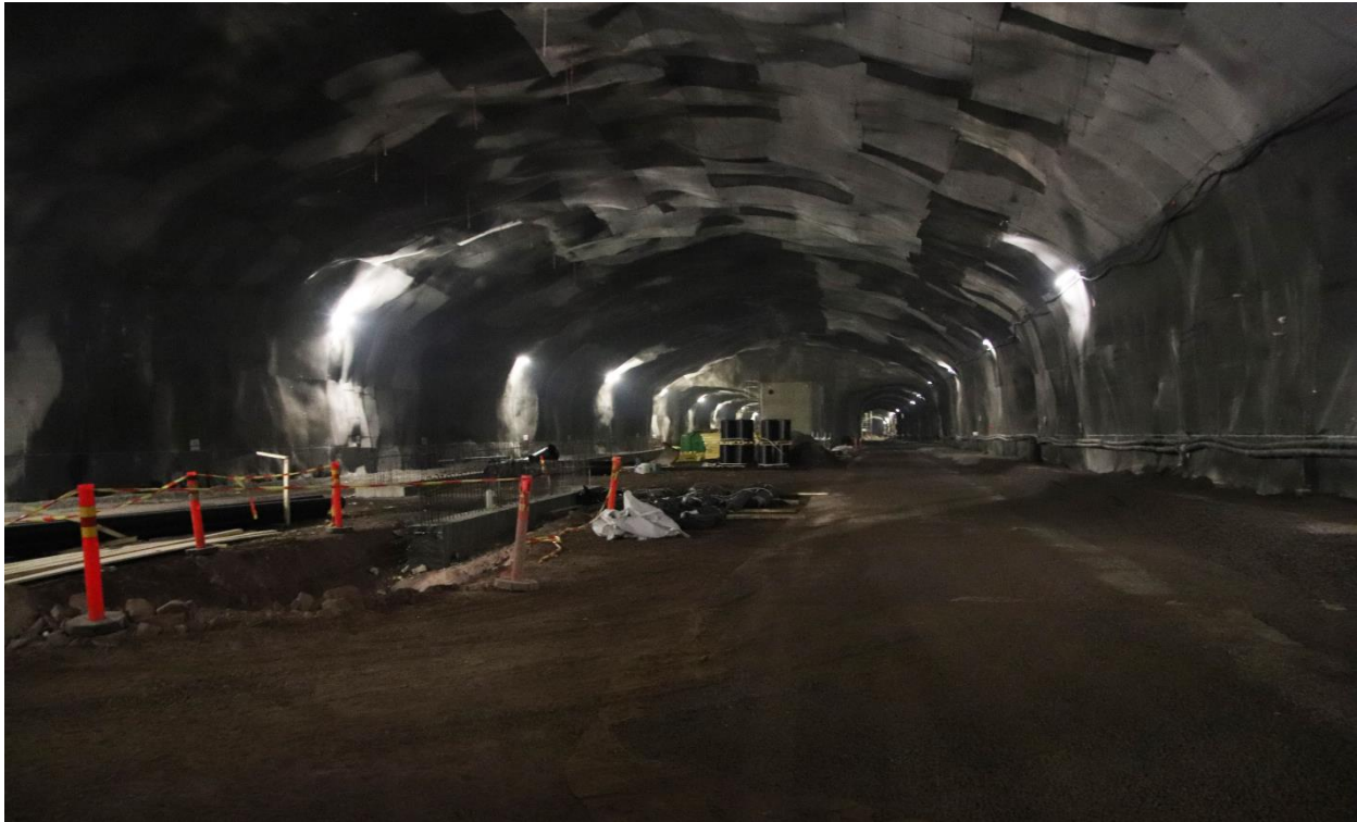
Tunneling works being completed at Kivenlahti station (photo courtesy Länsimetro)
