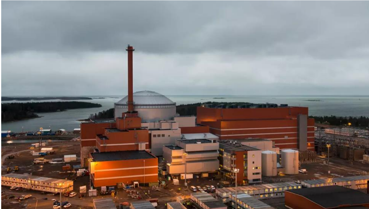
Olkiluoto 3 almost complete (photo courtesy Hannu Huovila / TVO)
