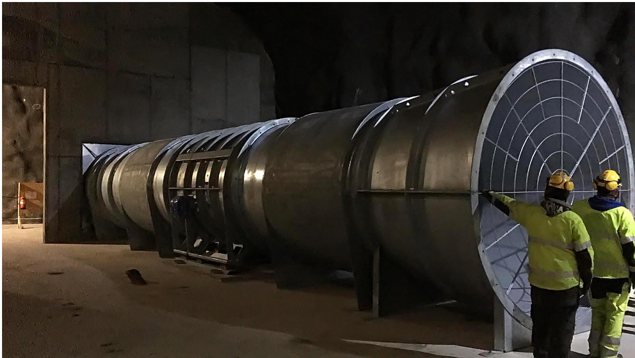
Installing smoke exhaust blowers at Espoonlahti station (photo courtesy R. Kaunismäki)
