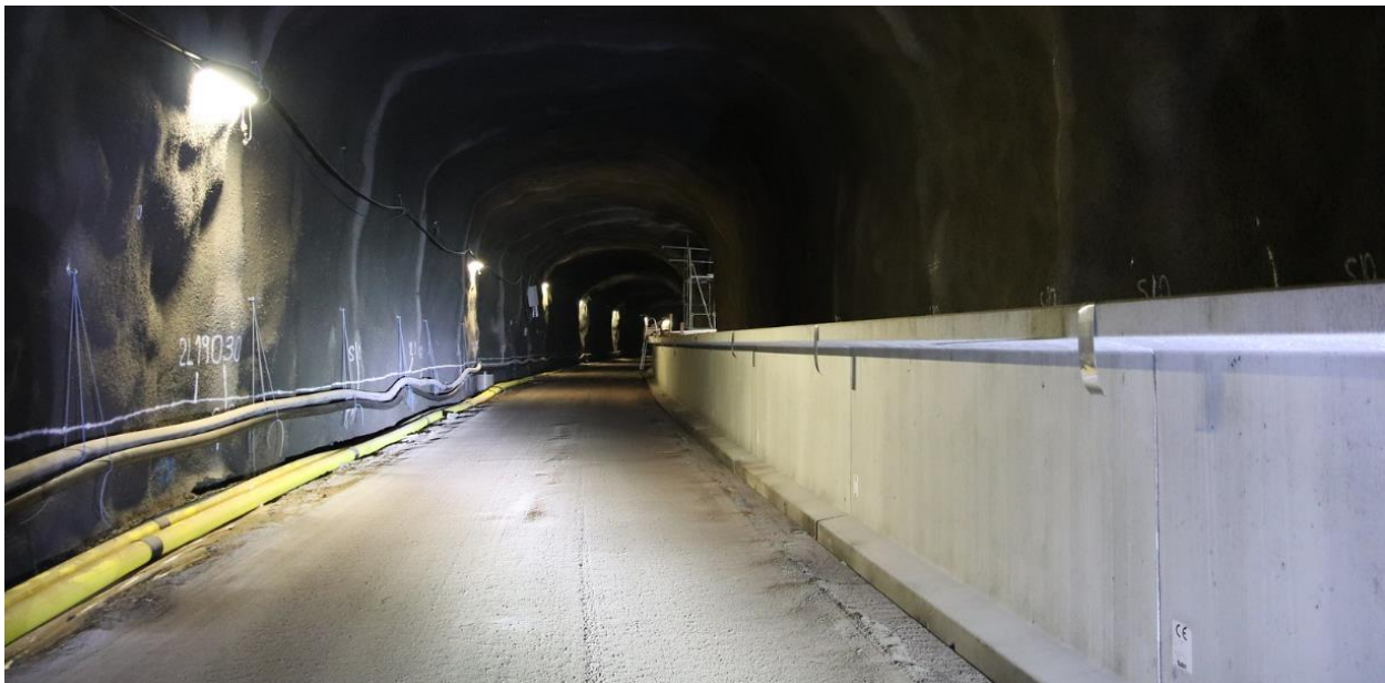
The track between Espoonlahti and Soukka stations (photo courtesy M. Wirman / Länsimetro)
