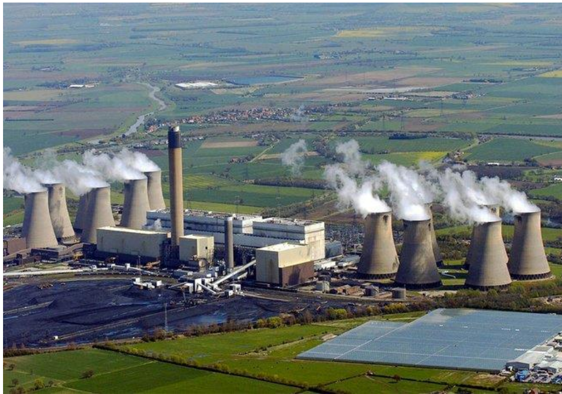
Drax Power Station (Image: Industry Europe)
