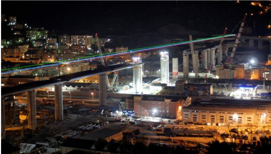
“Bridge of Light in Genoa”, courtesy of Salini Impregilo Group
