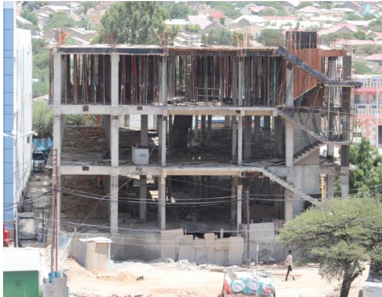
Figure 4: Photograph of an ongoing building construction project in Hargeisa
