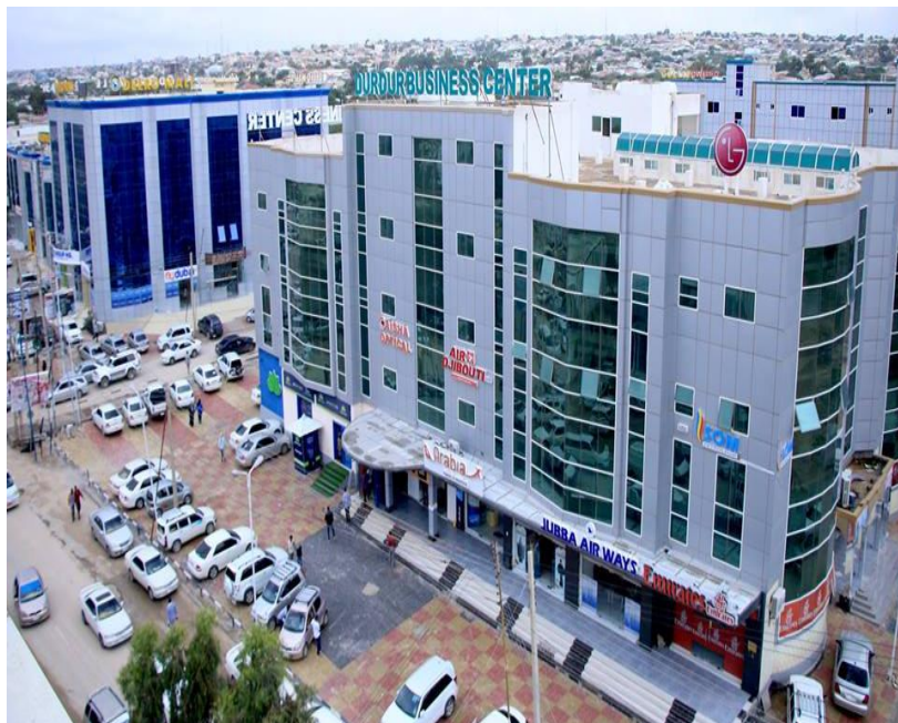
Figure 7: Photographs of some of the completed building construction projects (mix-use buildings) in Hargeisa
