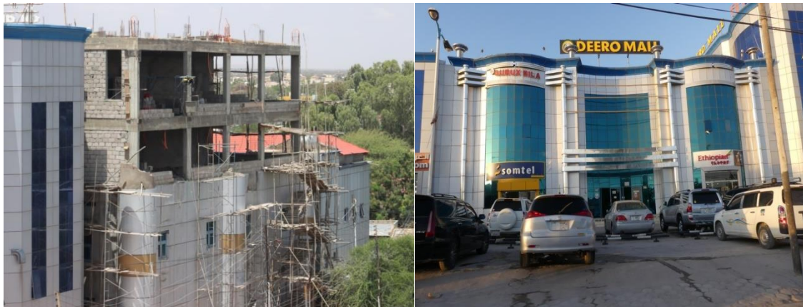
Figure 3: Photograph of building construction projects in Hargeisa
