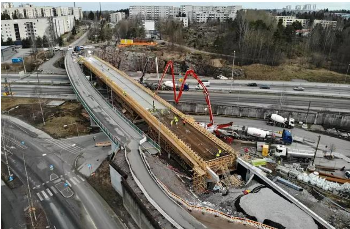
Raide-Jokeri bridge concrete pouring at Viikki (photo courtesy Jussi Laamanen / YIT)
