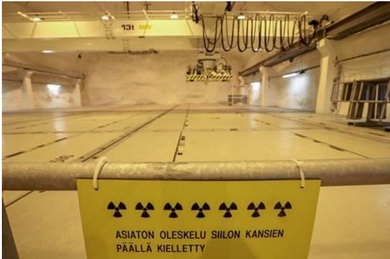
Olkiluoto 3 is nearing completion (photo courtesy Seppo Kärki / HS)
