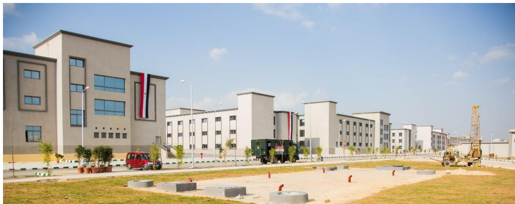
Figure 6. Tactic Village, the administrative building
