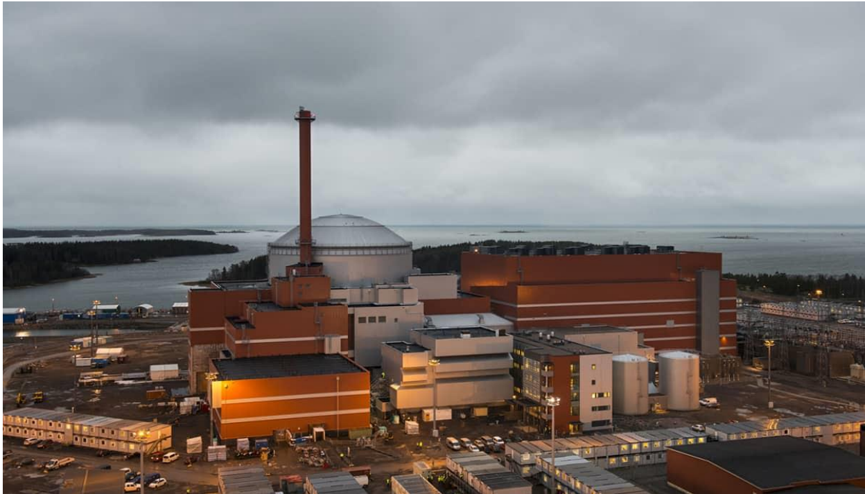
Olkiluoto 3 is nearing completion (photo courtesy Hannu Huovila / TVO)
