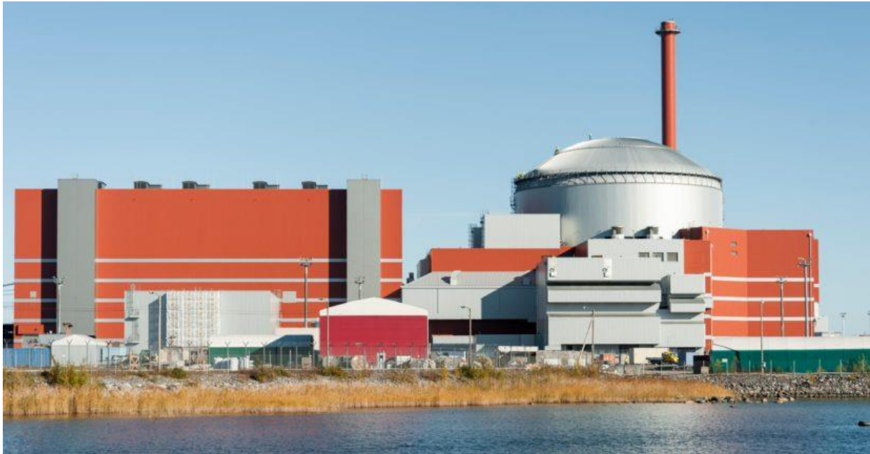
Olkiluoto 3, recovering from a number of setbacks, is nearing completion (photo courtesy TVO)
