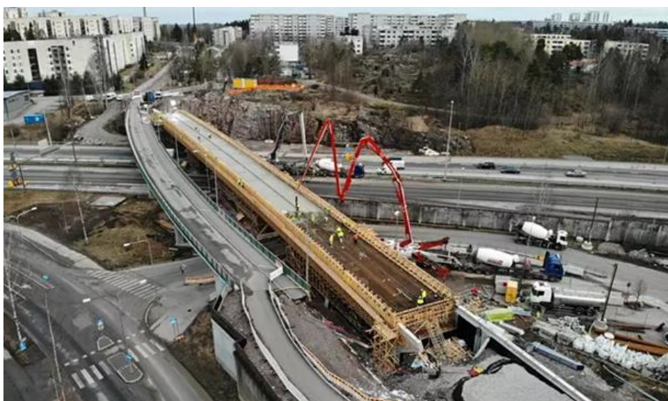
Raide-Jokeri bridge concrete pouring at Viikki (photo courtesy Jussi Laamanen / YIT)
