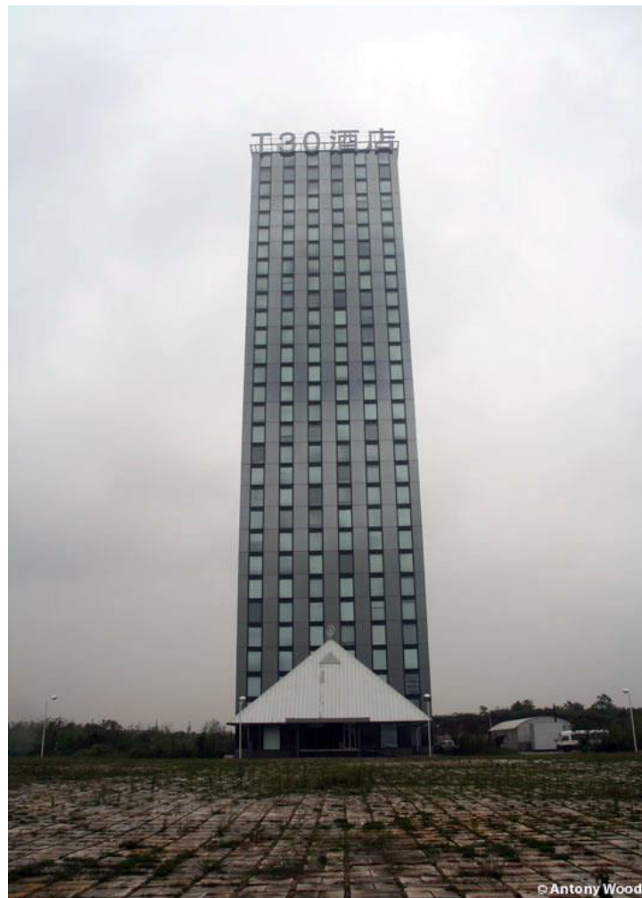
Fig.01: Completed T30 building in Huna Province, China 3
