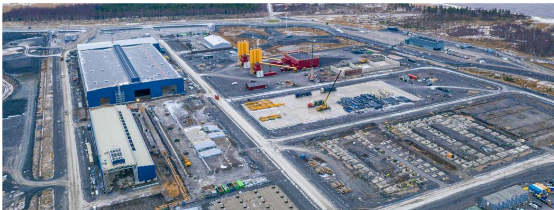
Hanhikivi1 construction site aerial view on 30.12.2020 (photo courtesy hanhikivi1.fi)
