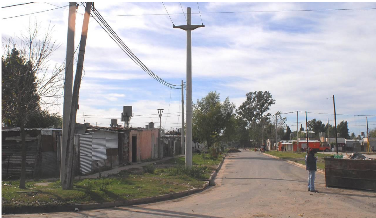
Empalme Project - After implementation of the Rosario Habitat Program
