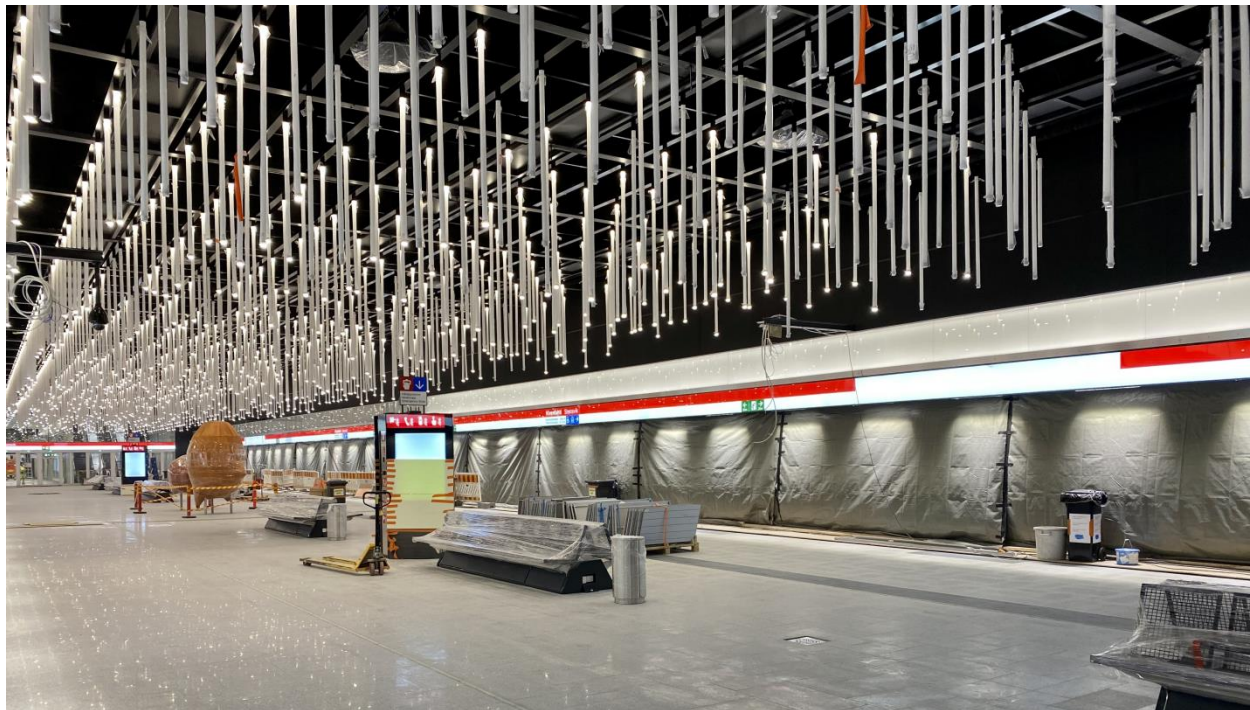
Kivenlahti metro station platform in April 2021 (photo courtesy Länsimetro)
