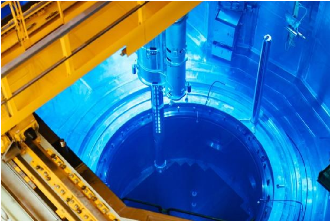
Nuclear fuel loading about to commence in Olkiluoto 3 reactor building (photo courtesy TVO)
