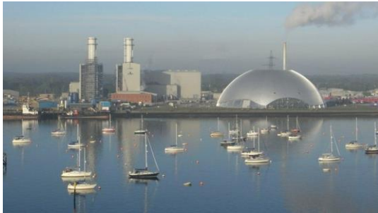
Marchwood Power Station (Image Chris Allen via BBC)
