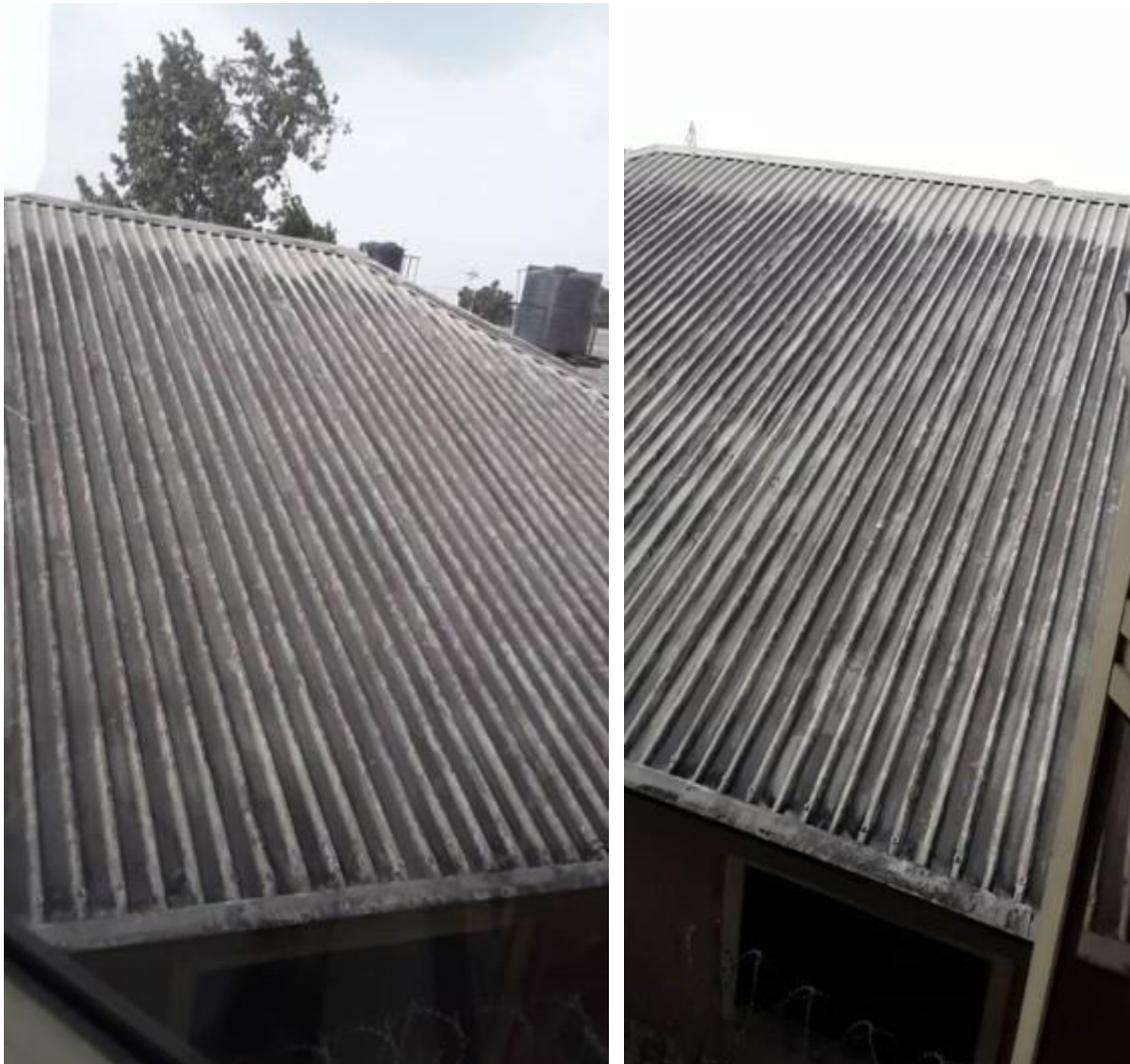
Figure 5 and 6: Black soot on the roof top of a residential building in Rivers State
