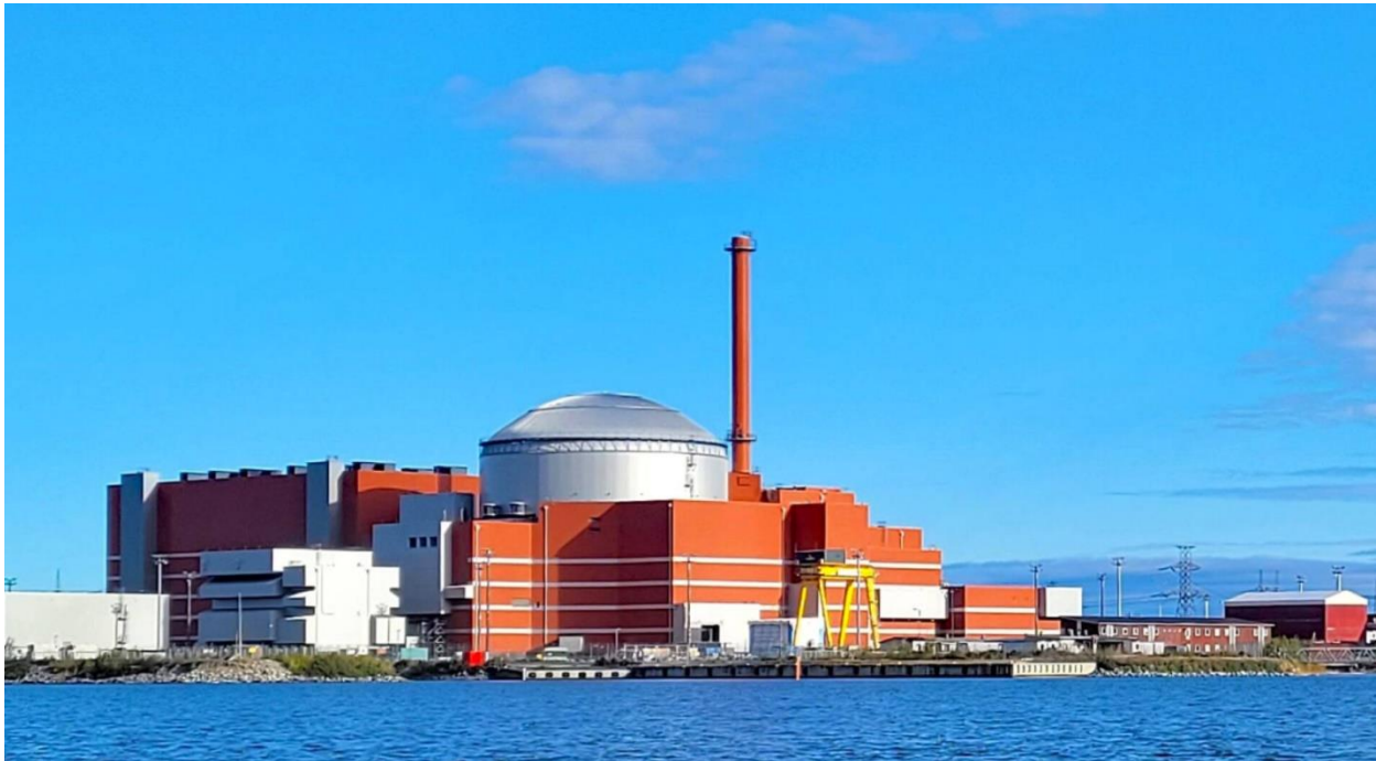
Olkiluoto 3 power station is now completed (photo courtesy Kari Suni / Sanoman Arkisto)
