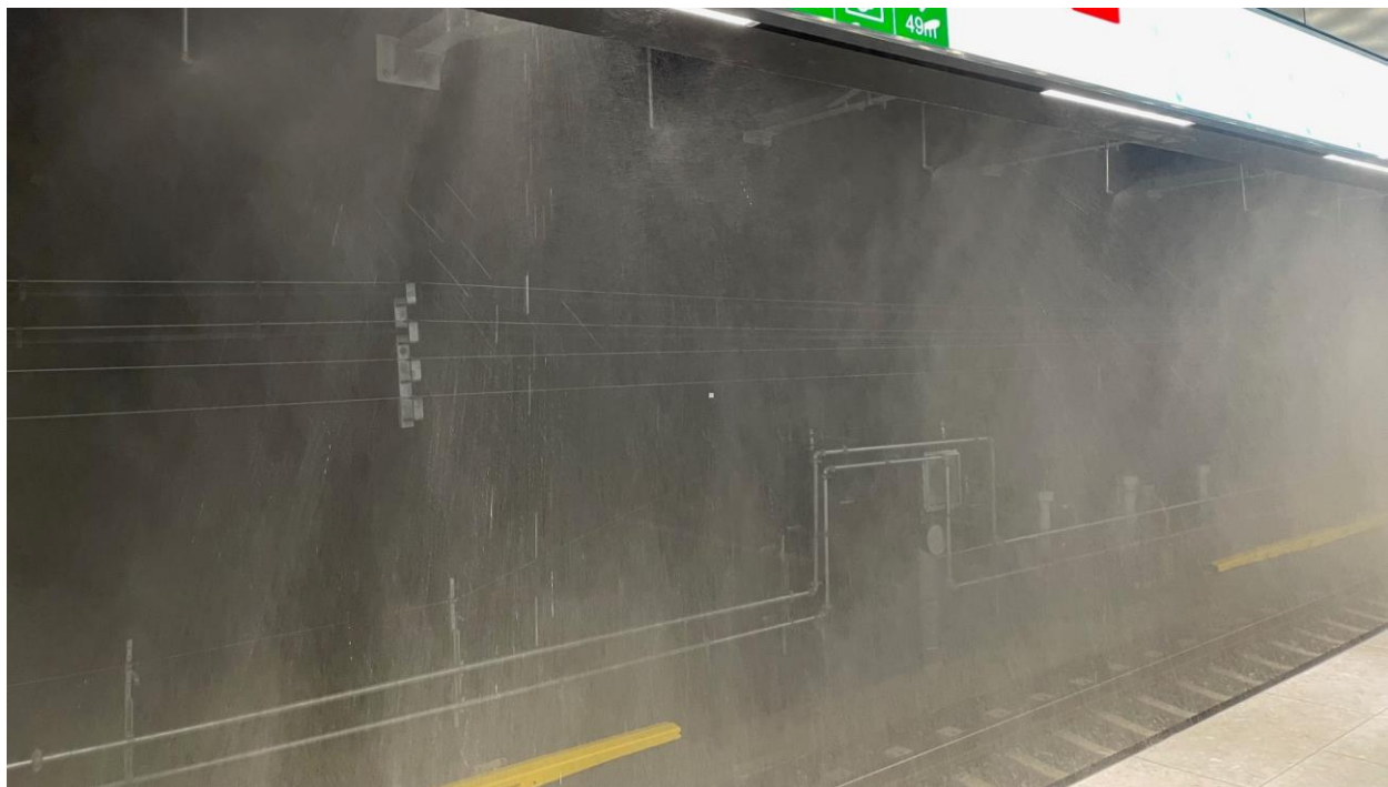
Special fire inspection at the Soukka metro station (photo courtesy www.lansimetro.fi )
