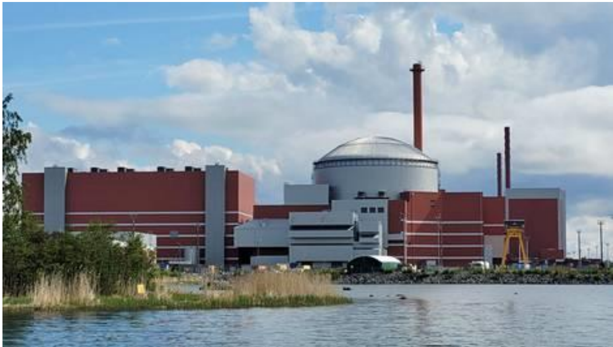
Olkiluoto 3 power station is now completed (photo courtesy Kari Suni)
