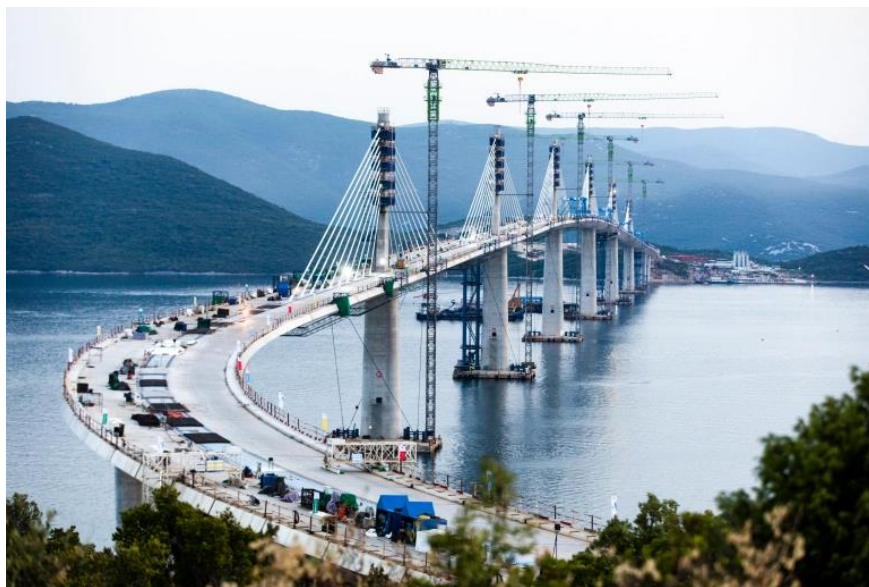
Peljesac Bridge under construction
