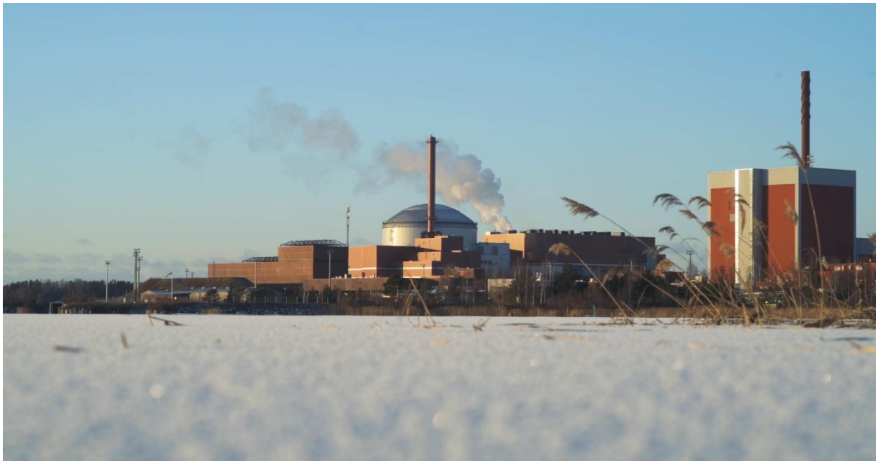
Olkiluoto 3 and 2 power stations in winter weather (photo courtesy TVO)
