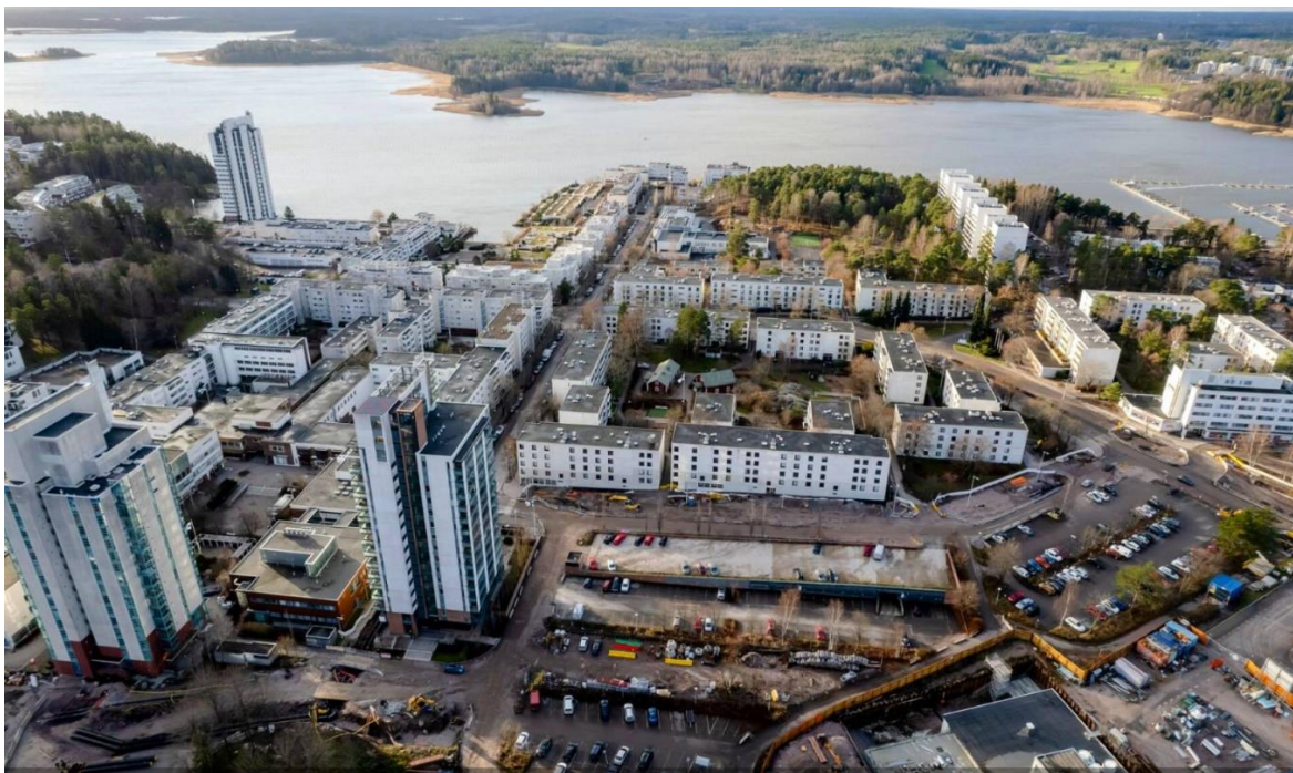
Aerial view of Kivenlahti, with the metro station construction site at the bottom (photo courtesy Kalle Koponen / HS)
