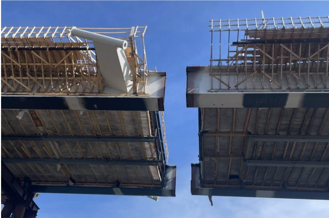
The Kruunuvuorensilta bridge deck is now almost completed (photo courtesy kruunusillat.fi)
