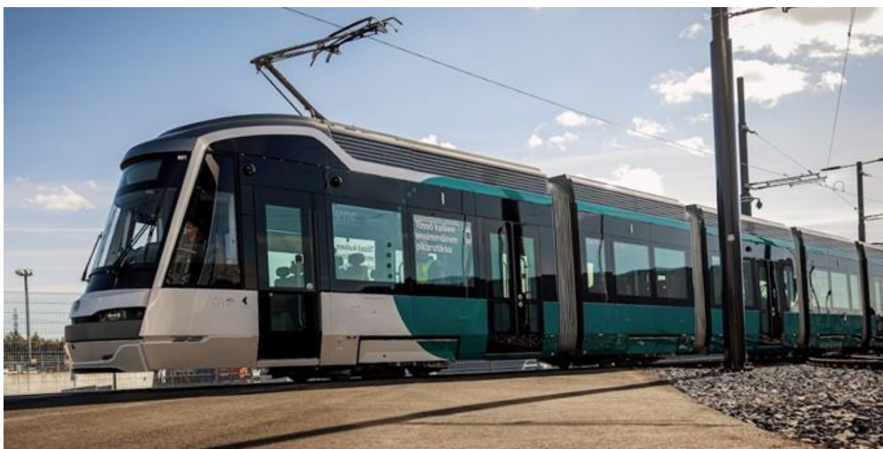
Raide-Jokeri light rail line is now fully operational (photo courtesy Raide-Jokeri project)
