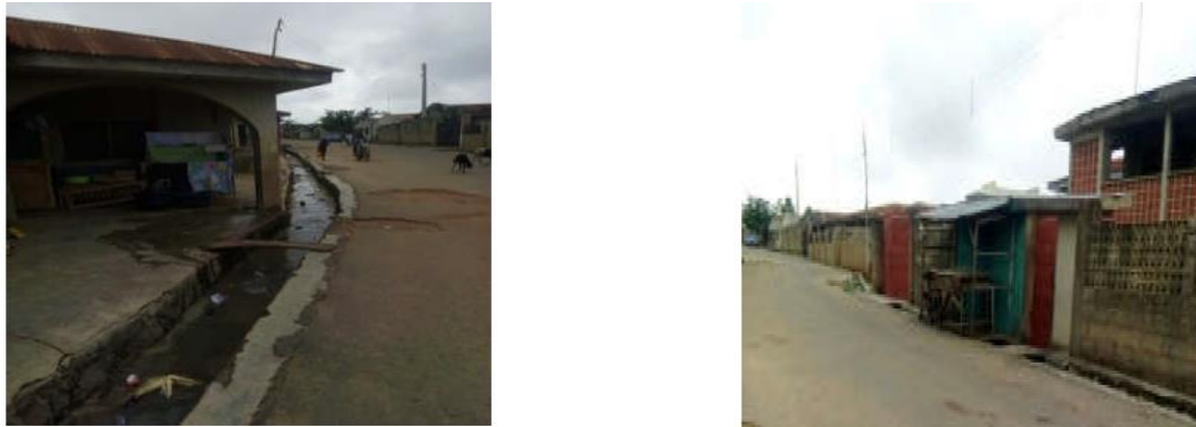
Figure 5: Residential Building along Olubose Street, Ajegunle area of Oyo.
