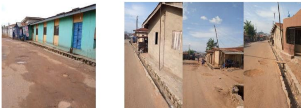
Figure 6: Residential Building along Olubose street, Ajegunle area of Oyo
