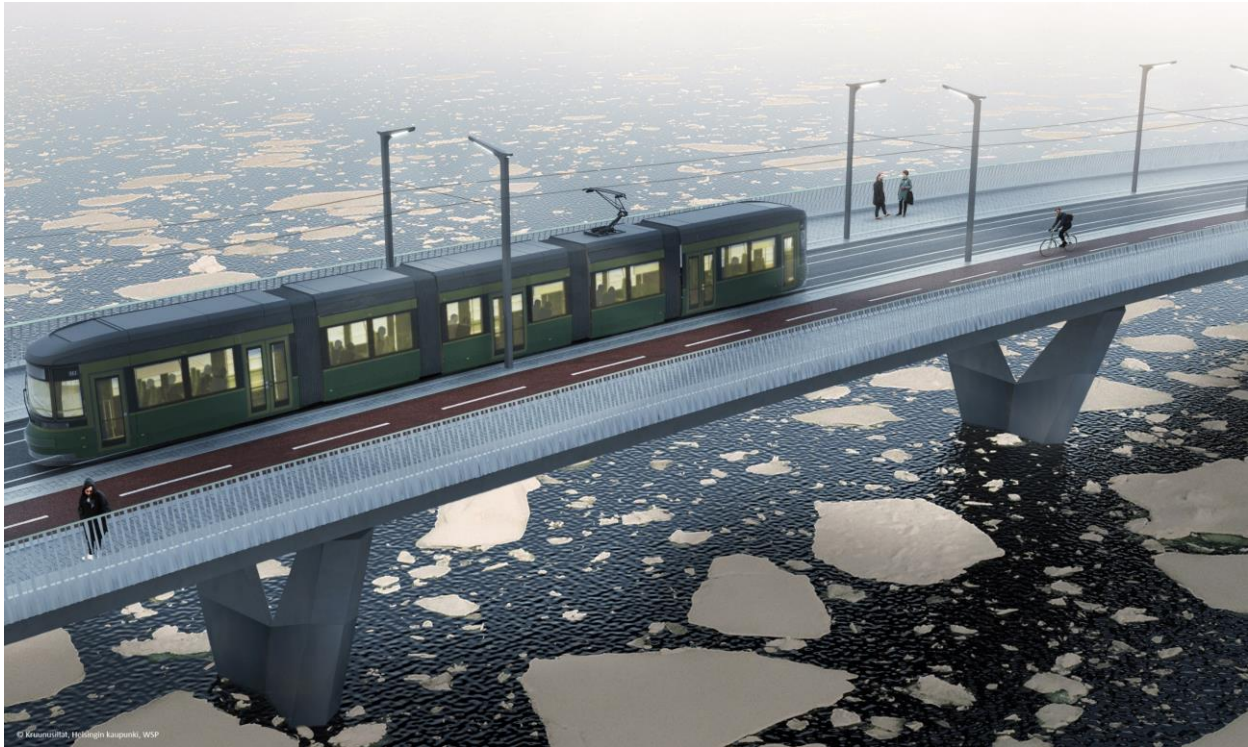
Artist's view of Kruunuvuorensilta from in spring (illustration courtesy Kruunusillat, City of Helsinki, WSP)
