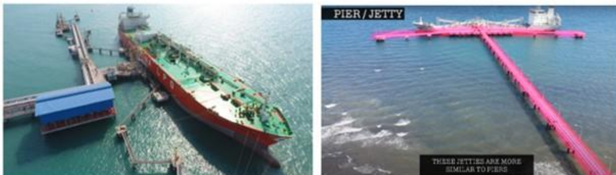
Figure 3-Typical Mooring Dolphin Jetty 5, 6
