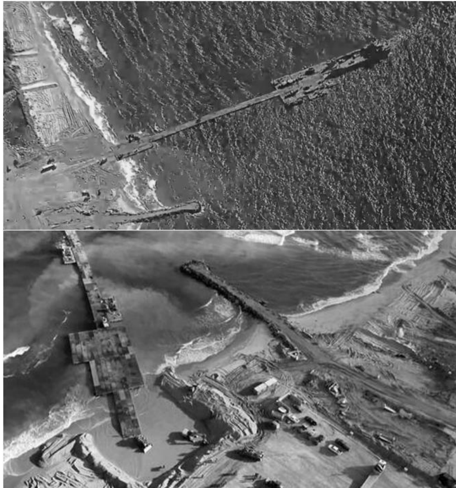
Figure 32. Pier Reassembled After Being Damaged
