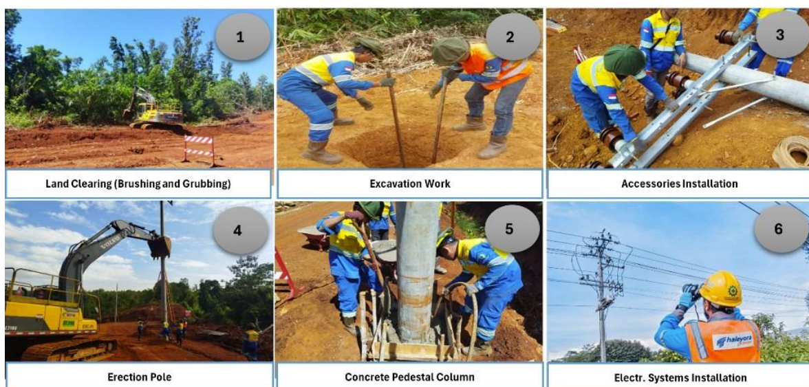
Figure 3. Work Sequence Construction 1000kVa Overhead Electrical Power Distribution Line
