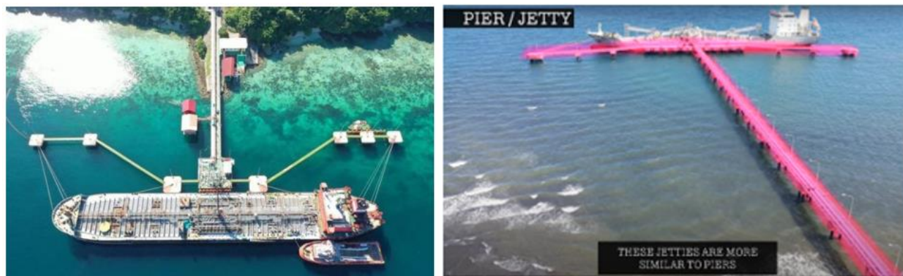
Figure 2 Typical Dolphin Pier/Jetty used in Pertamina Patra Niaga 9 10
