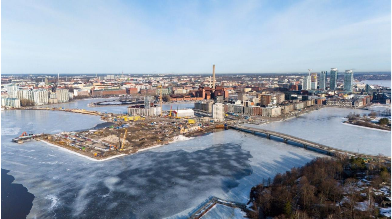
Aerial view of Merihaansilta (left) and Finkensilta (right) (photo courtesy Sami Kero / HS)
