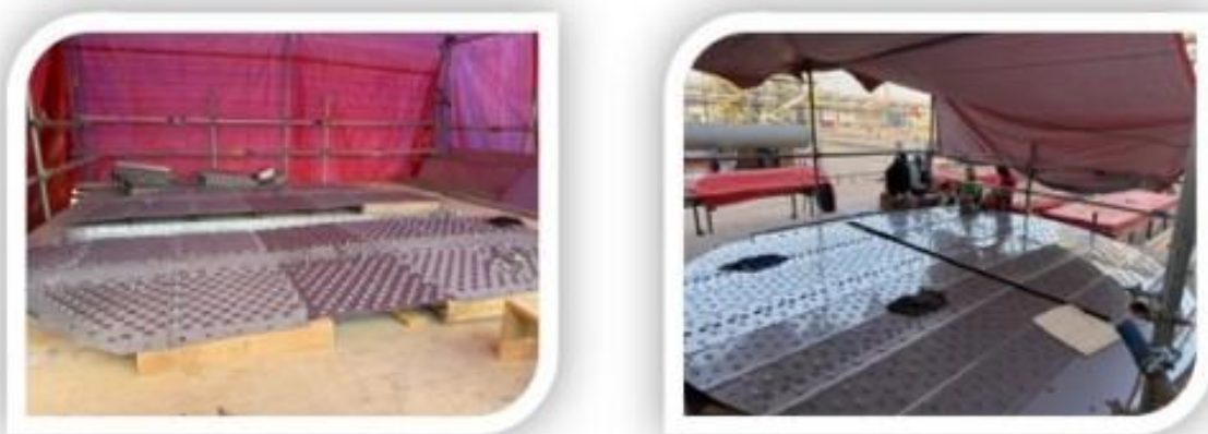
Figure 5: Tray Pre-Assembling
