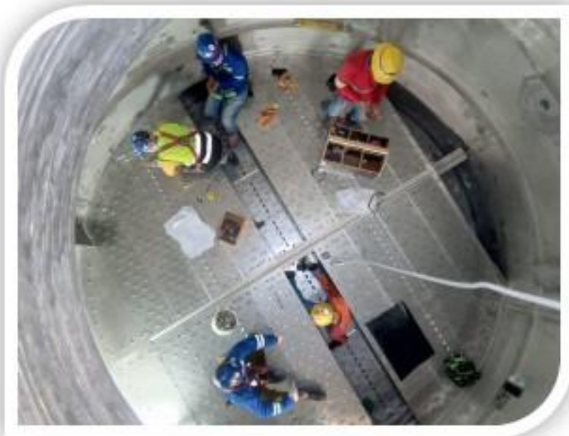
Figure 7: Tray Installation
